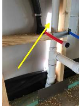
Visible gap in the WRB sheathing
