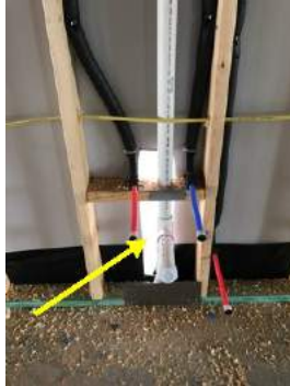
Visible gap in the WRB sheathing
