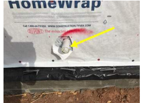
Tape around pipe penetration
