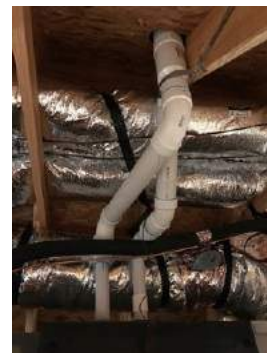
HVAC flue ok
