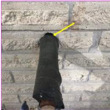
Seal wall penetration (font facade)
