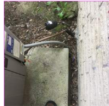
Missing insulation
