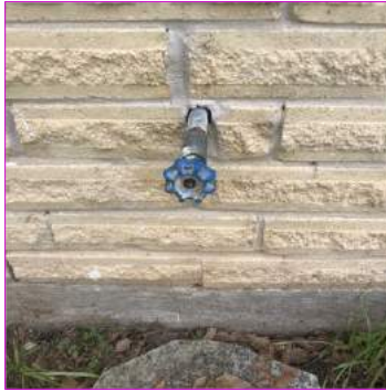
Seal wall penetration (back facade)
