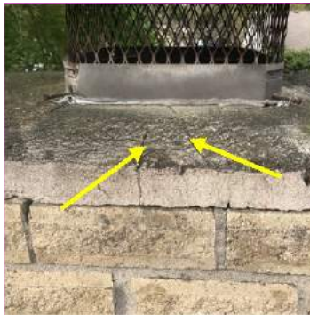
Moderate cracks
