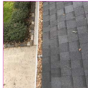
Gutter debris
