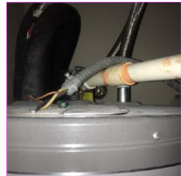
Exposed wires
