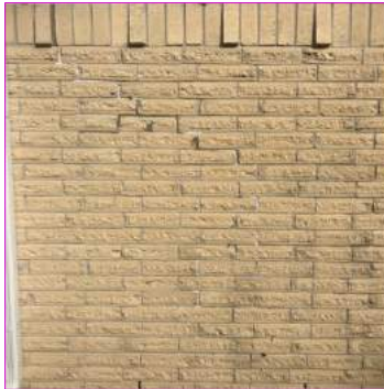
Repaired step cracking (left facade)
